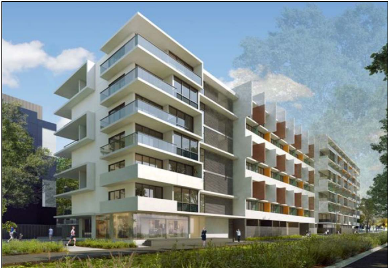
Figure 13: View of Buildings B and E looking north along Joynton Avenue
