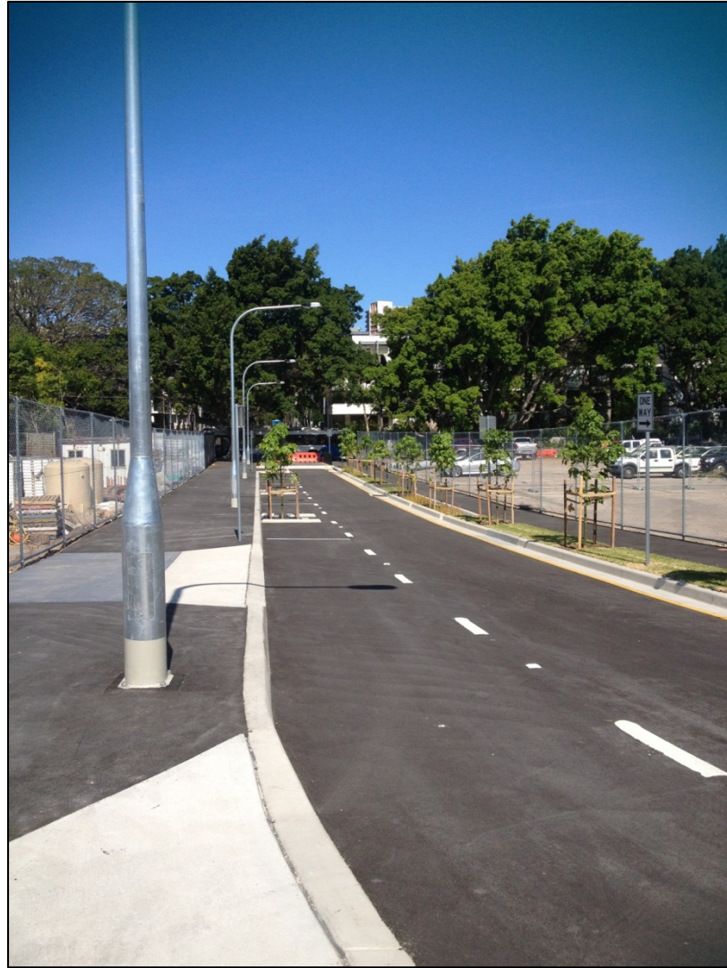
Figure 3: The completed Lamond Lane that connects Joynton Avenue to Merton Street
