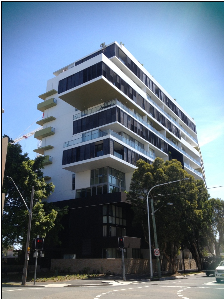
Figure 2: The completed Stage 1 building (known as Building G) as viewed from the corner of O'Dea Avenue and Joynton Avenue
